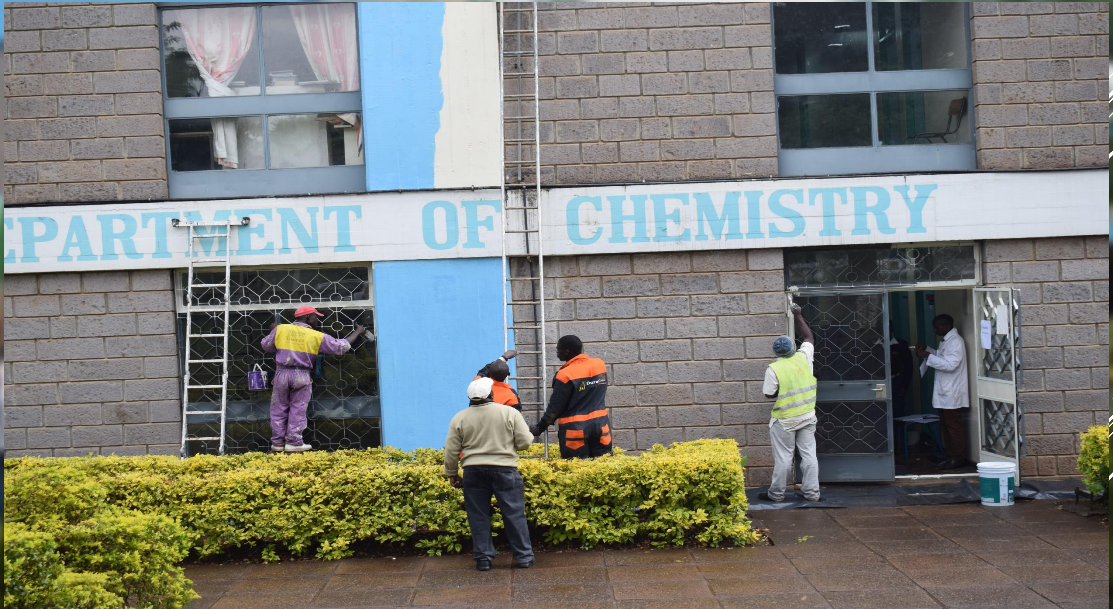
Painting the Exterior Walls of the Department of Chemistry using Lead Free Paints Donated by Basco Paints Company
